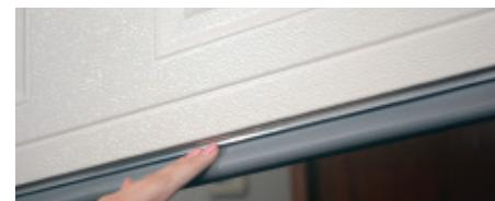
Hörmann minimizes floor corrosion by utilizing an aluminum bottom seal retainer that never rusts and is more durable than brittle plastic retainers.
